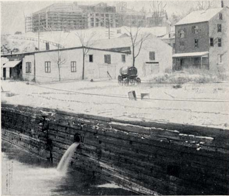
The increase of population brings with it an increase in the amount of sewage which we do not realize until we see the size and number of sewer outfalls pouring their contents into the river
