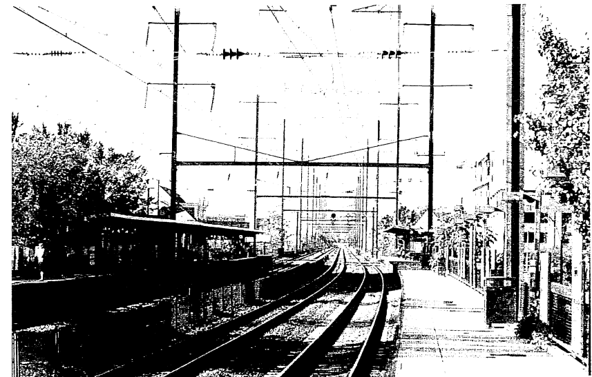
Electrified Railroad Through New Brunswick, 2008
