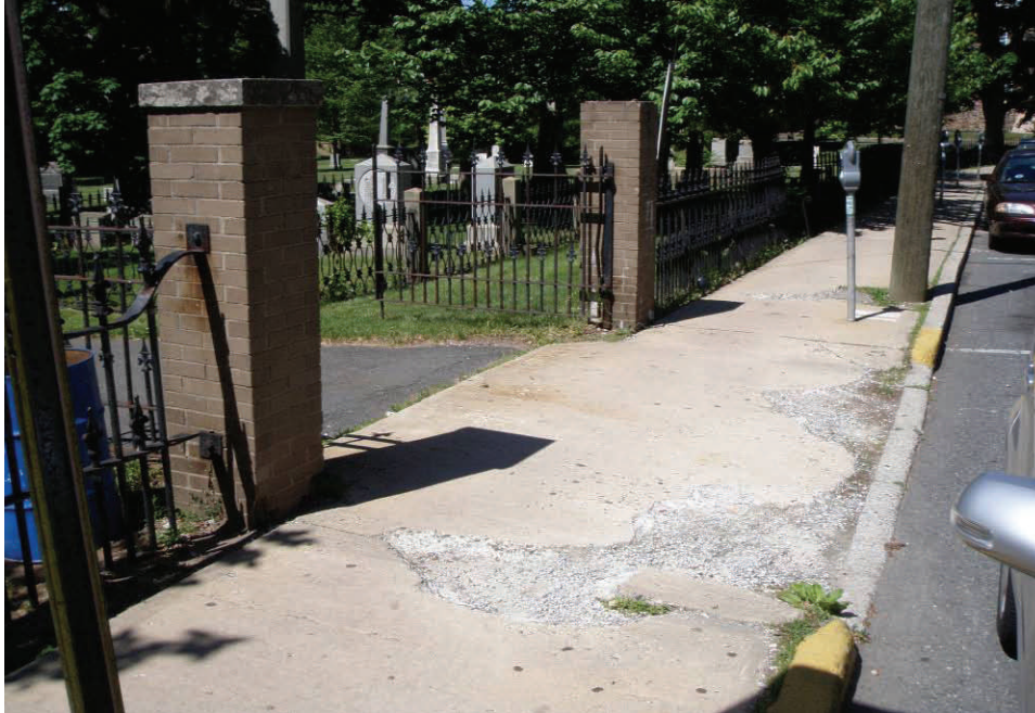
Photo 1: North border on Morris Street. Note the poor condition of the public sidewalk.
