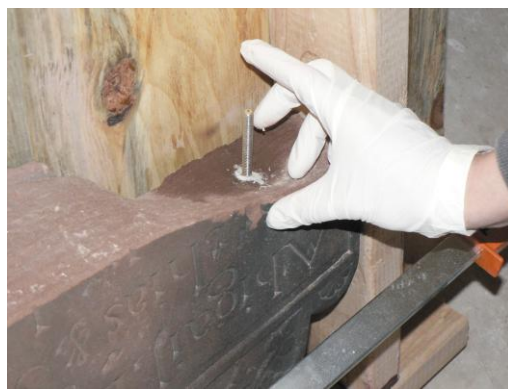
Treatment: Typical installation of pins (not this site – First Presbyterian Church of Elizabeth, NJ, 2007).
