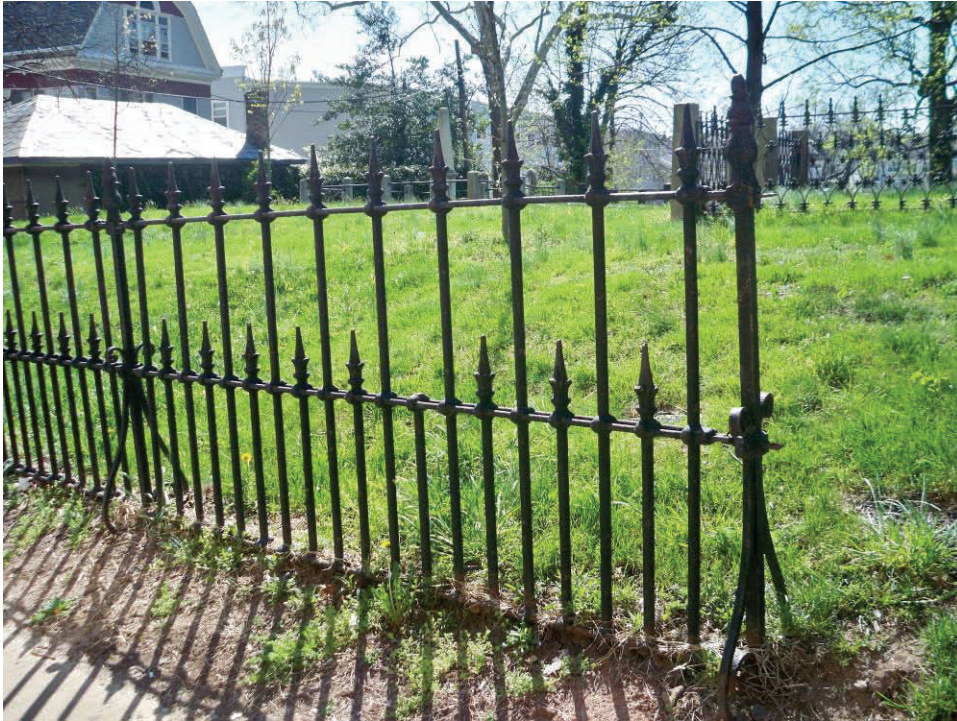
Photo 26: A typical section of the Presbyterian and Cheesman section fencing. Note that the grade is above the base rail. In this section, the problem seems to be coming from the site.
