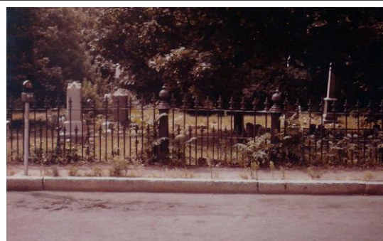
Ca. 1972 disrepair, provided by Connolly & Hickey Historical Architects.
