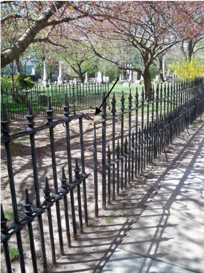
Photo 26: A typical section of the Presbyterian and Cheesman section fencing. Note that the grade is above the base rail. In this section, the problem seems to be coming from the site.
