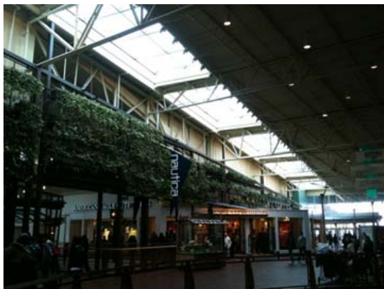
Jersey Gardens Mall, Elizabeth, New Jersey
