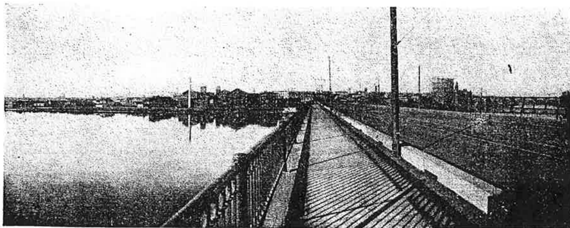
VIEW OF CITY FROM ALBANY STREET BRIDGE
