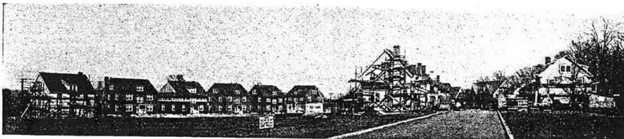
GROUP OF HOMES BEING ERRECTED IN HIGHLAND PARK
