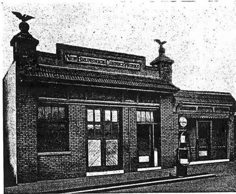
OFFICE AND WORKS, JELIN STREET
