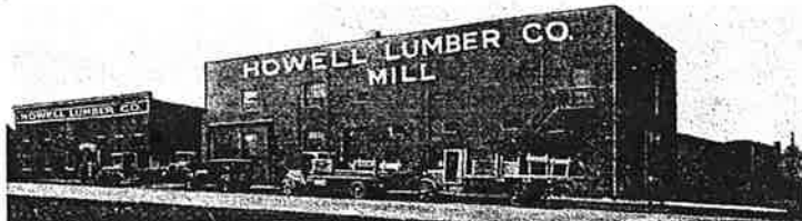
UPTOWN OFFICE YARD AND MILL
